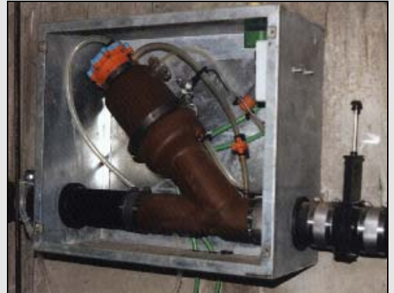
Interface Valve mounted in wall cabinet
