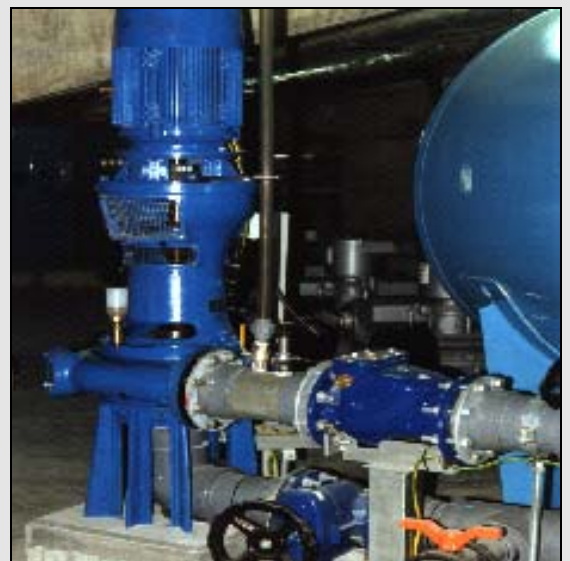
Discharge Pump and Pipework
