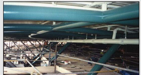
Vacuum ring main suspended from roof structure.
