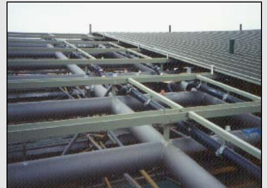
Black PE vacuum pipes visible in roof prior to cladding
