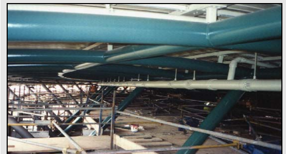
Vacuum ring main suspended from roof structure.
