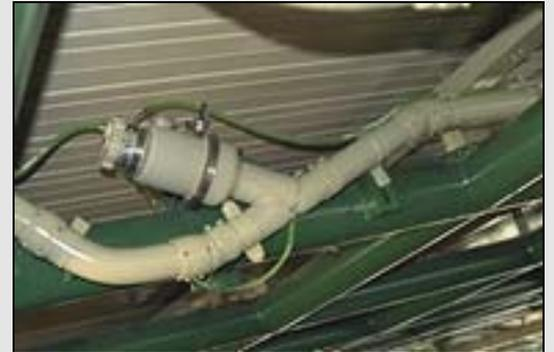
Iseki Vacuum Interface valve suspended in roof
