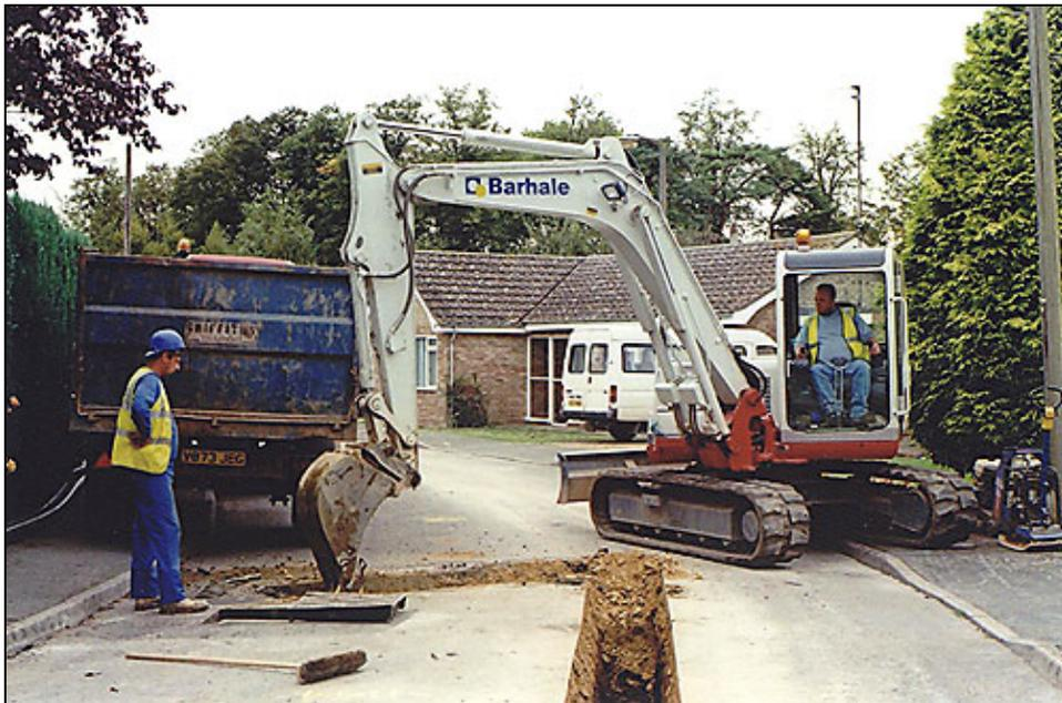
Completed in August 2003, the residents of Gorefield are now served by a state of the art sewer system which greatly reduces any potential impact on the environment. The installations, comprising of 5000m of polyethylene sewers and 105 vacuum interface valves, were completed with very little inconvenience to the residents and minimum disruption to local road traffic and businesses.
