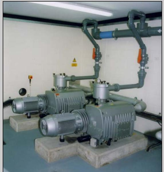
630m<sup>3</sup>/hr vacuum pumps installed
