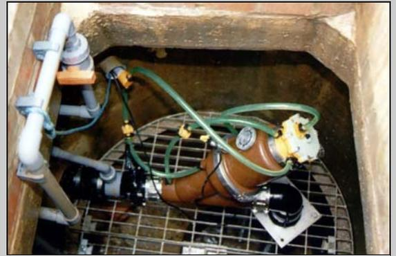
Iseki Redivac Interface Valve installed in chamber
