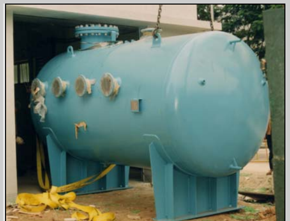
Vacuum vessel being installed
