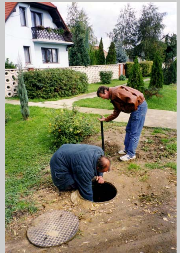
Valve Chamber Inspection
