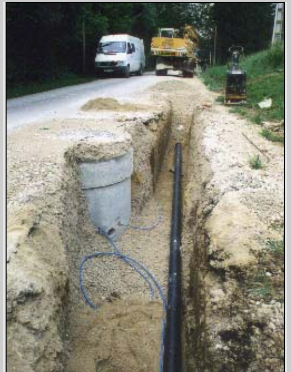
Trench with vacuum pipe, valve chamber and monitoring cable
