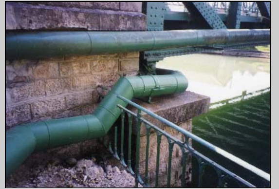
Vacuum sewer attached to the bridge abutment
